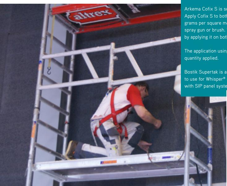
Arkema Cofix S is supplied in a canister of 25lt or about 20 kg. Apply Cofix S to both corresponding surfaces at a rate of 200 grams per square metre. Adhesive may be applied to surfaces with spray gun or brush. This is sufficient to cover 40-50 m² of coverage by applying it on both bonding faces as a contact adhesive.
